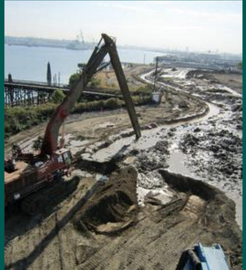
Contractors at the Arkema cleanup site dig an underground wall meant to prevent contaminated groundwater from leaking into the Willamette River. Department of Environmental Quality
